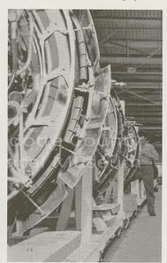
Engines for B-25's go through final inspection and preparation before being hoisted and fitted into place in wing nacelles.
